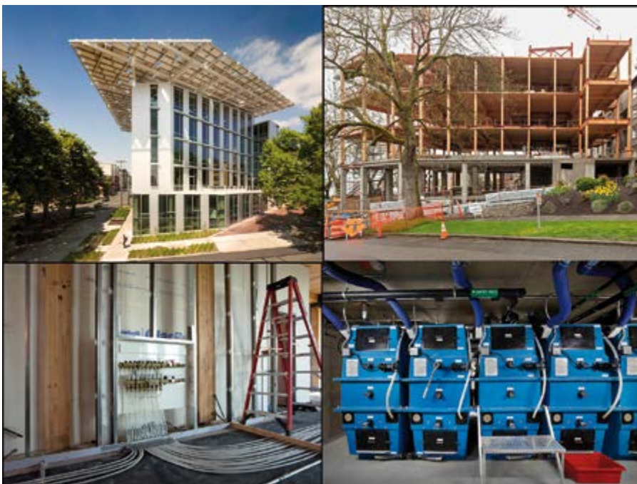
Fig 8. The Bullitt Center Building. General edification view (photo by John Stamets); wood pillars structure during the construction; hydronic heater controller and composters (photos by Brad Kahn). [Source: flickr/bullitt_center | Creative commons CC BY-NC 2.0)
